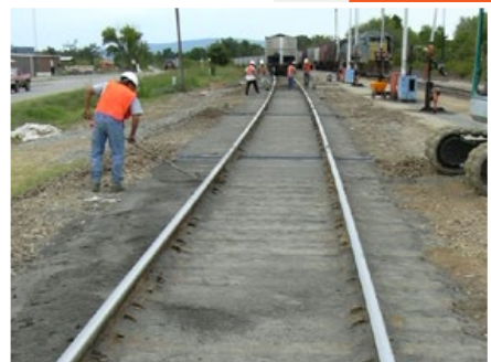
Crossdrain Install and Site Prep
